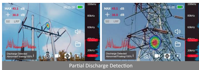
Partial Discharge Detection
